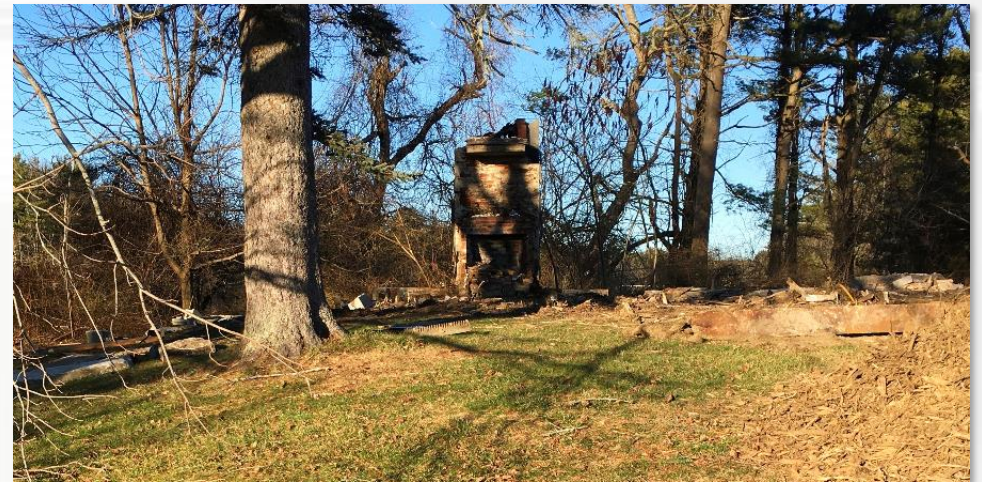
The living room fireplace midway through demolition
