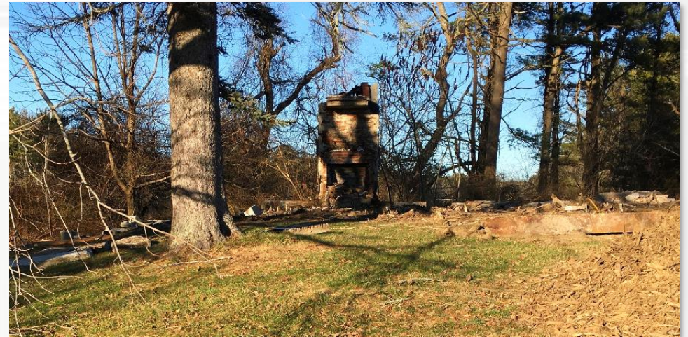
The living room fireplace midway through demolition
